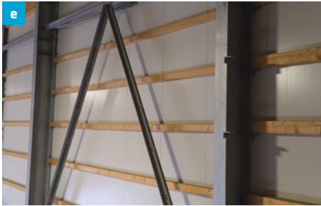
The enclosure of the pre-treatment line seen from the outside.
